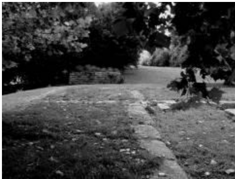
Remaining Shaker Landing building foundations.
