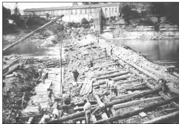
Rebuilding Dam No. 4 at Frankfort in 1885.
