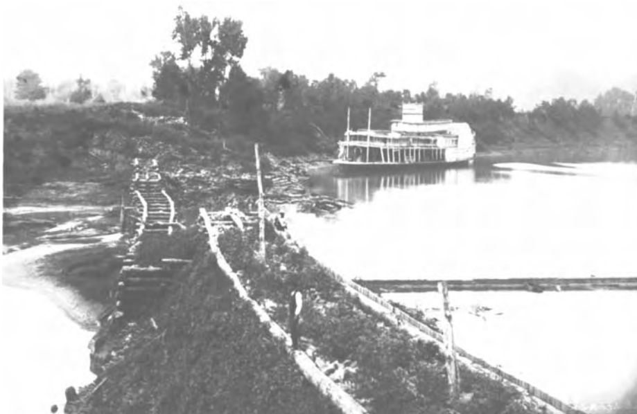
Deteriorated conditions at Dam No. 1 during the 1870's, with steamboat United States in the background.
