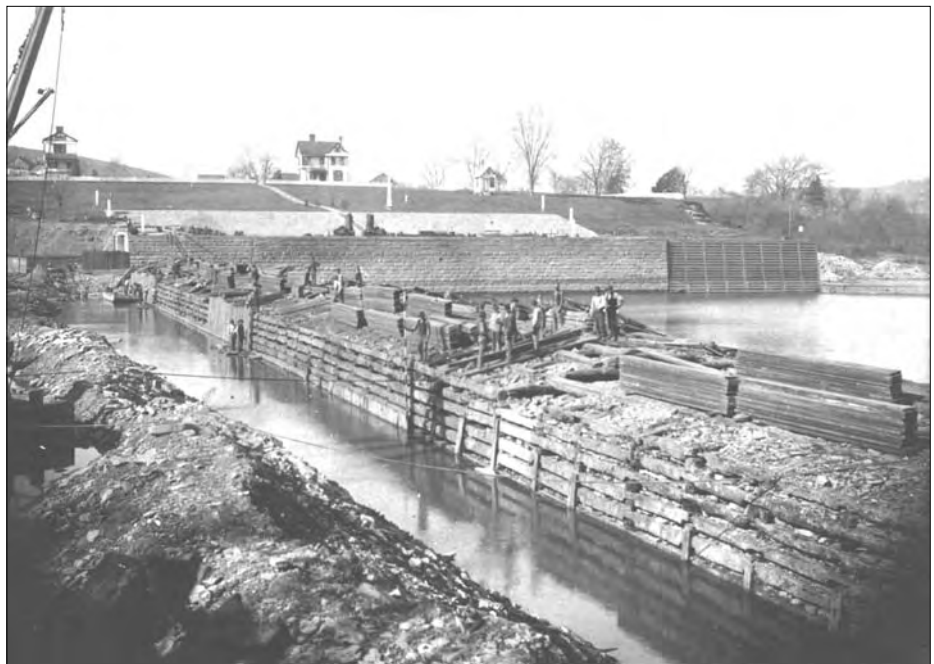
Timbercrib dams were constructed by framing pens resembling log cabins, setting them side by side across the river, then filling them with stone and planking the top.
