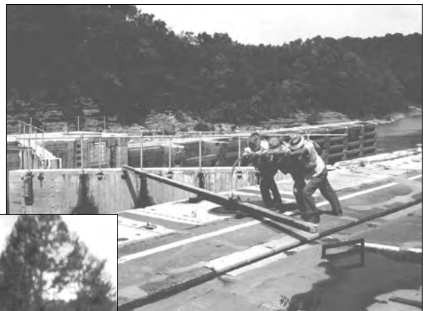
Lockmen turn the capstan to open the gates at Lock No. 8. In addition to turning the capstan in circles, they walked up and down the lockwalls to each capstan.
