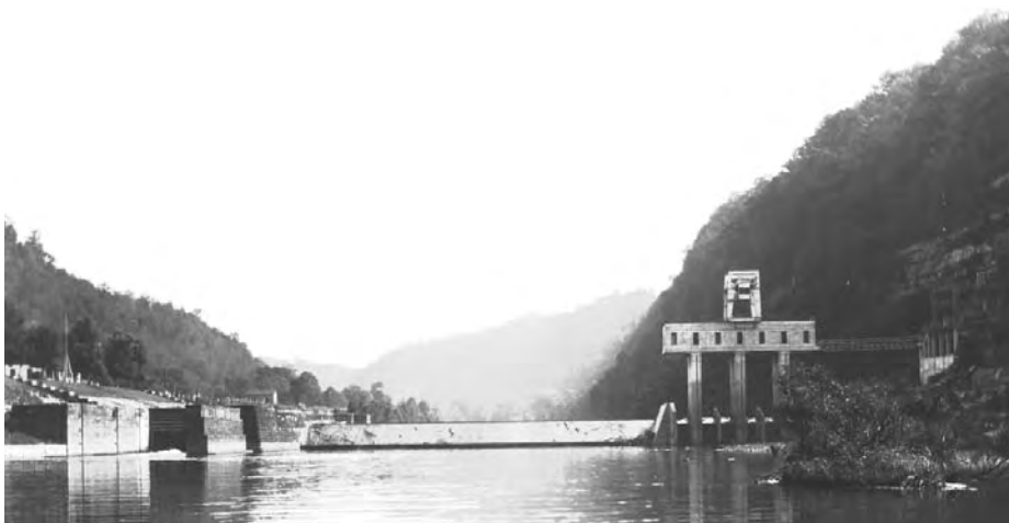
No water passed over Dam No. 7 during the 1930 drought. Structure on the right is the Kentucky Utilities powerhouse.
