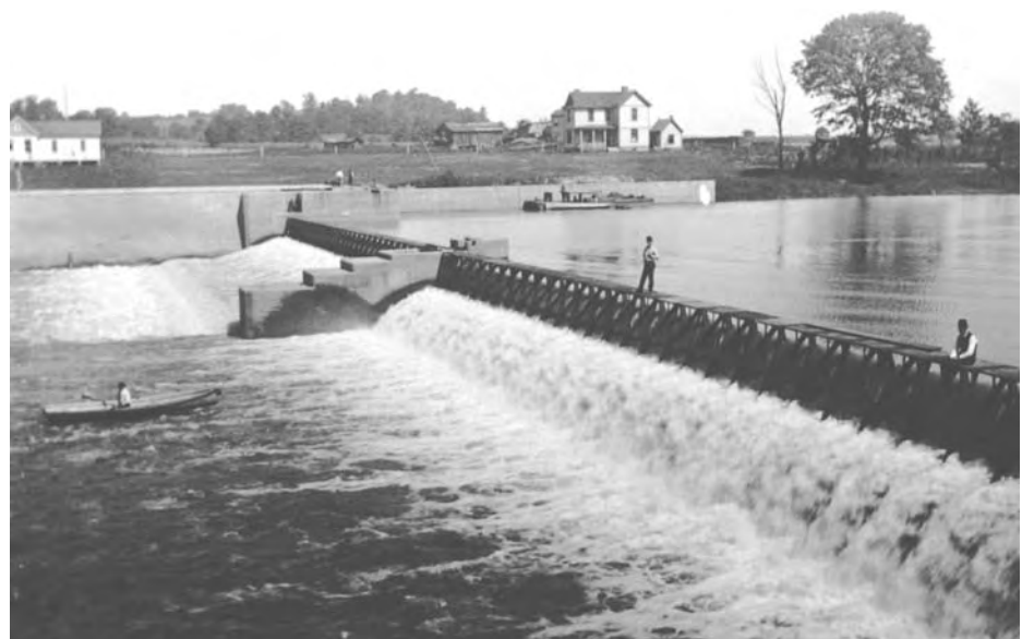
Movable crest and walkway across the dam are in place in this view.
