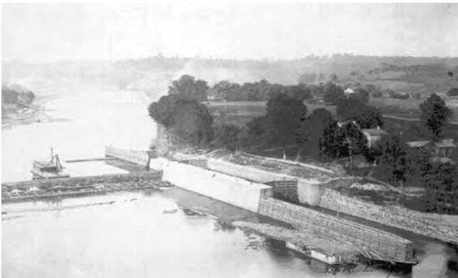
Plans for the Kentucky River project included navigation locks of stone masonry and dams built of timber cribs filled with stone.
