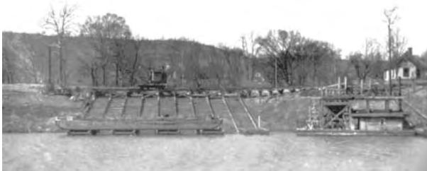
Launching a barge at marineway adjacent to the Frankfort repair yard at Lock No. 4 in 1923.
