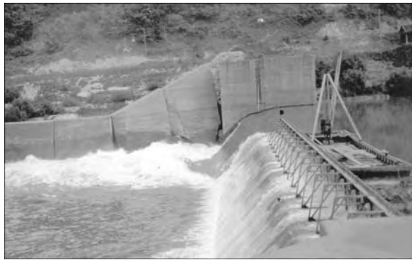
The maneuverboat is lowering the movable crest atop Dam No. 13 because the river is rising.
