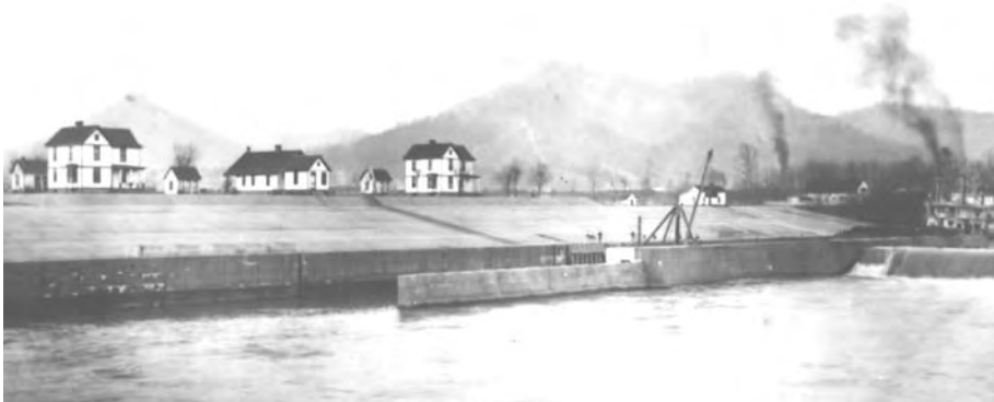
Lock and Dam No. 12 completed. Note the three lockhouses, provided because operating the movable dam crest required a crew of three men.
