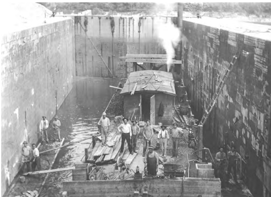
Workers make repairs inside a Kentucky River lock.
