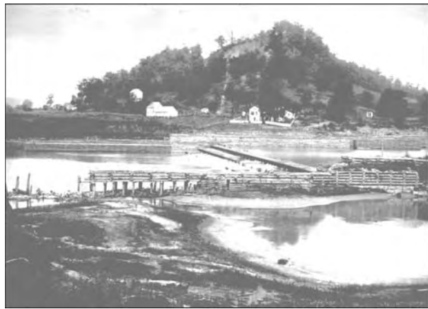
View of the breached Dam No. 1 near Carrollton in 1883.
