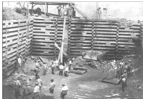
Men shovel muck inside a cofferdam into skips for hoisting and removal while a steam pump in the background removes the water.
