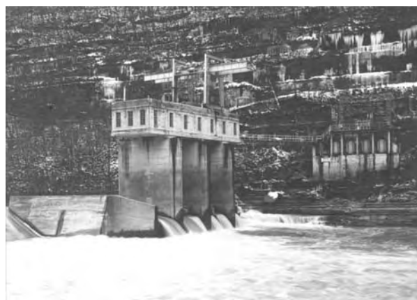
Kentucky Utilities powerhouse and transformer platform built at Lock and Dam No. 7 during the 1920s.
