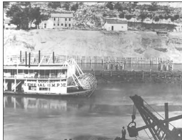
Snagboat General O. M. Poe and a dipper dredge working at Lock No. 7.
