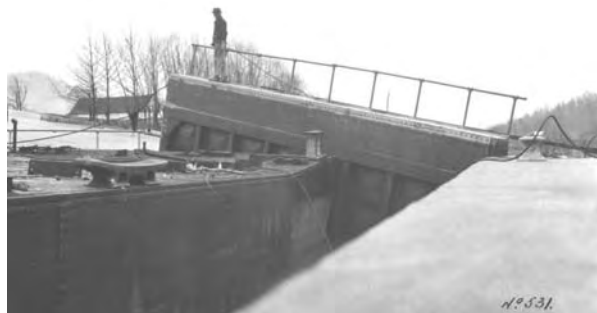
A barge towed by the Plymouth accidentally lifted a lockgate at No. 12 in March 1925.
