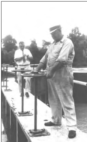
Operating valves in the lockgates was done by hand.
