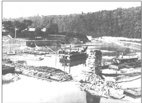
Rebuilding Dam No. 5 in 1885.
