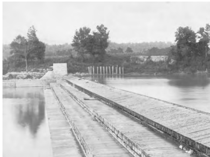
The finished timbercrib dams were planked over and stepped down like a staircase.
