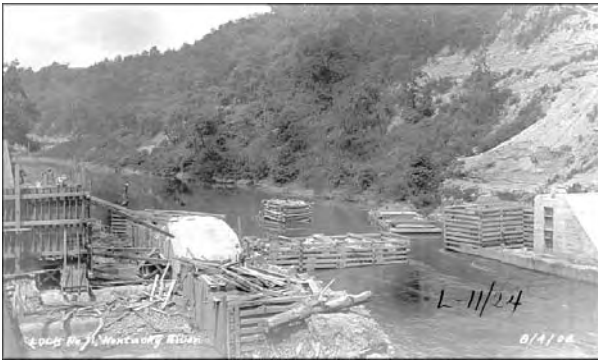
Floating timbercribs into place at a Kentucky River dam, 1906.
