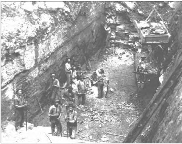
Excavation at Lock No. 7 in 1895 was still done with shovels and wheelbarrels.
