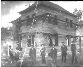
Lock house under construction for the resident lock keeper (lockmaster) and his family.
