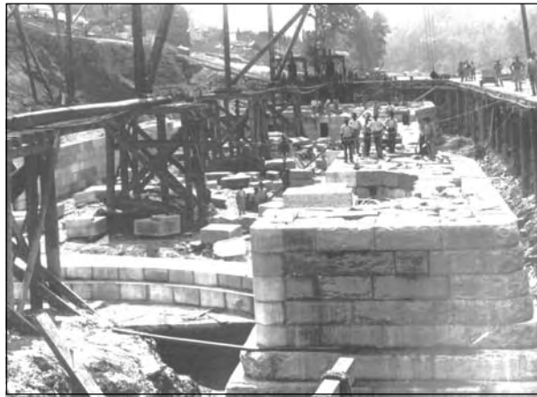
The Kentucky River navigation locks were built of stone masonry before 1900.
