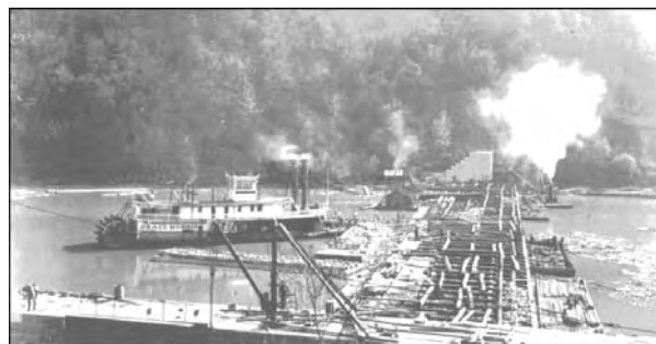
The steamboat Grace Morris assists with the construction of a timbercrib dam.
